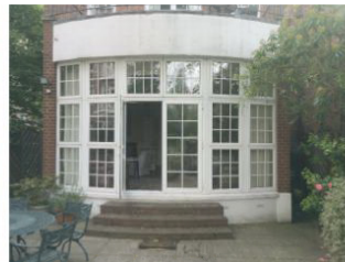
View from rear patio to existing lounge room
